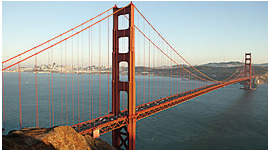
Golden Gate Bridge from Marin County looking at San Francisco
